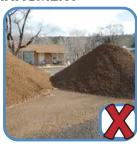
**Reduce or Eliminate Stormwater Contact with Material Piles -** Protect stockpiled materials from contact with stormwater with perimeter controls and covers such as secured tarps, silt fences and wattles.
