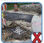
**Prevent Sediment and Debris from Entering the Storm Sewer -** Use temporary filter devices such as gravel bags, wattles, filter fabric or inlets inserts at storm drains and curb inlets to prevent sediment and debris from entering the storm sewer by filtering runoff. With proper erosion and sediment controls on the construction site, inlet protection is a your last line of defense to keep sediment out of the stormwater system.
