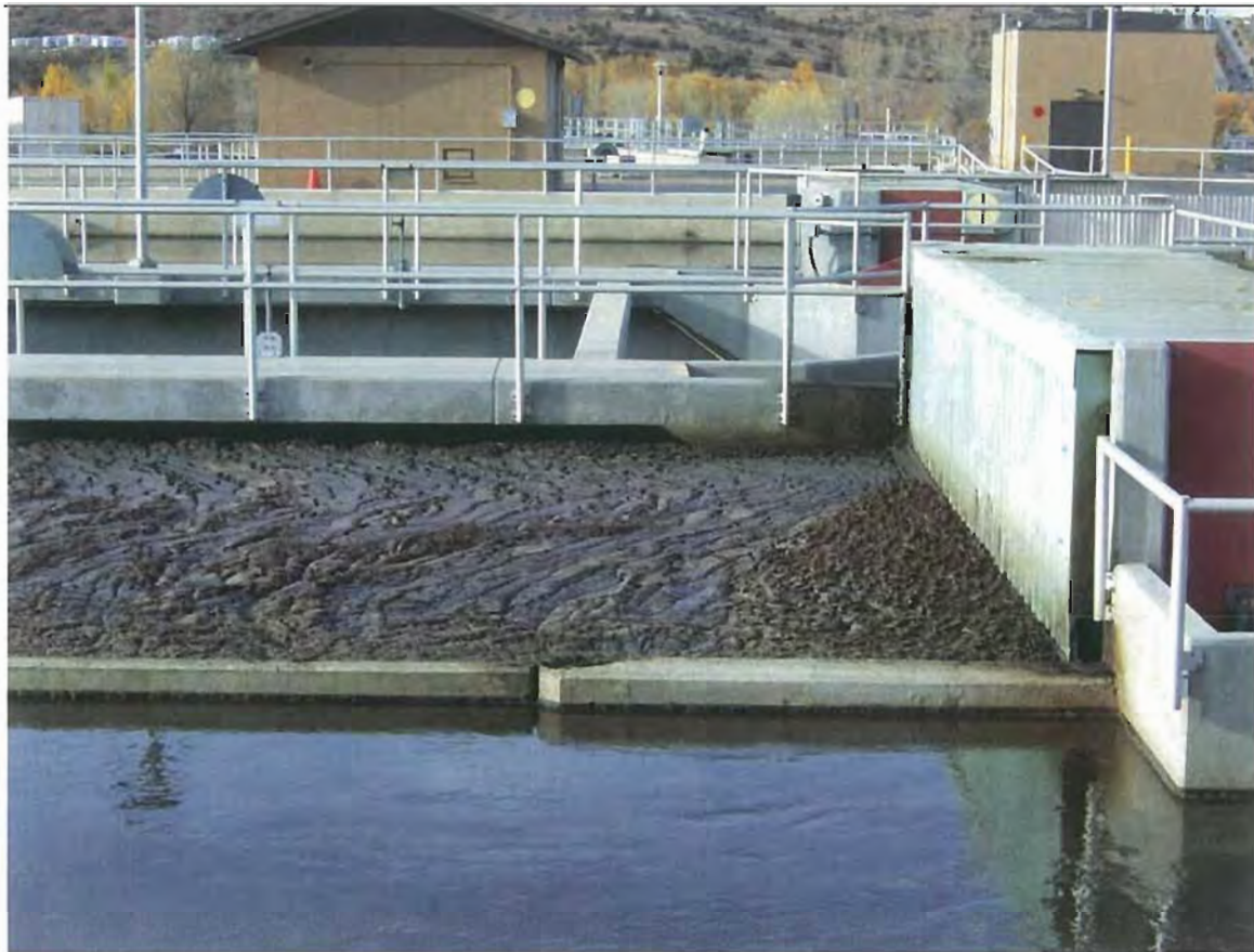
Figure 3-3 Filamentous Foam on Oxidation Ditches
