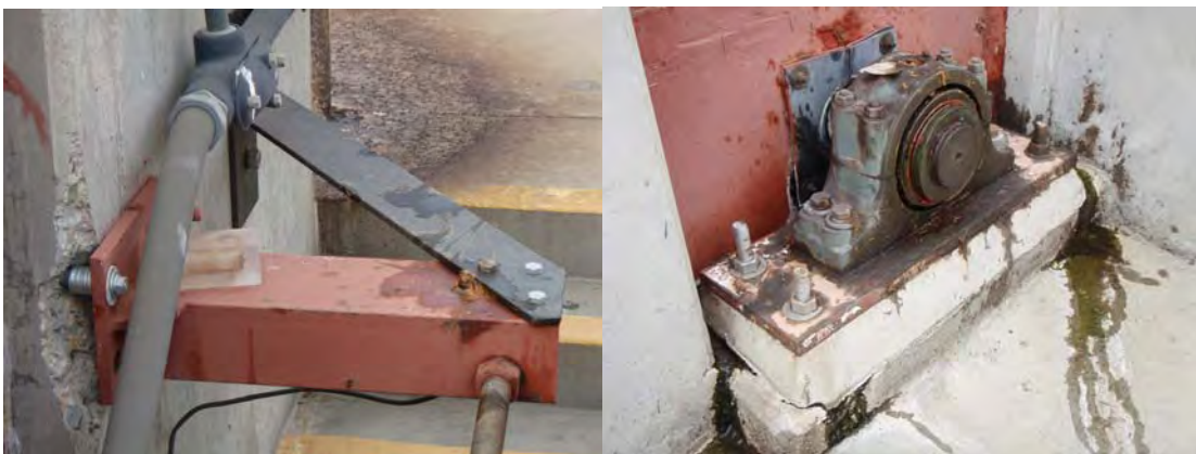
Figure 3.2 Oxidation Ditch Concrete Failures
