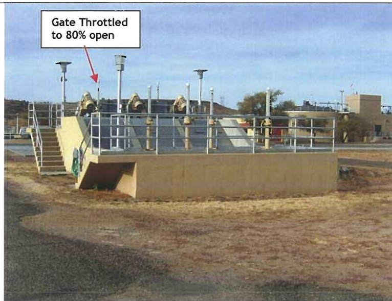
Figure 2-7 Sundog WWTP Flow Splitter
