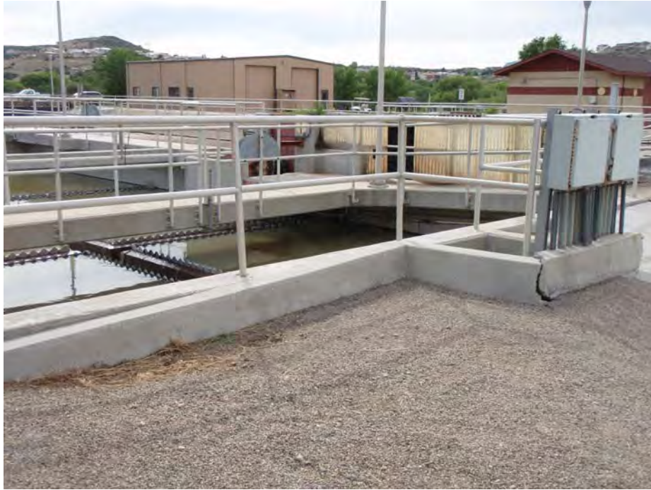
Figure 3.1 Settlement Along NE Corner of Oxidation Ditch
