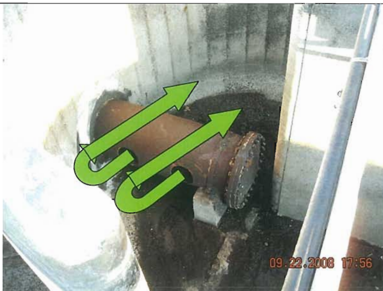
Figure 3-2 Ditch Inner Ring Influent Flow Distributor
