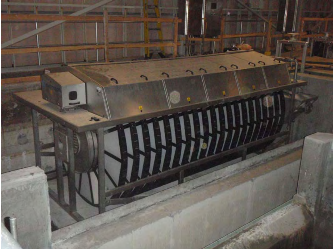
Figure 5.2: Kruger Hydrotech Disk Filter under Construction – Flagstaff, Arizona
