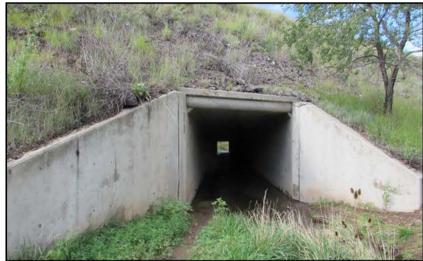
Figure 2. Existing SR 69 concrete box culvert located at MP 294.1, through which mule deer passage can be increased with barrier/funnel fencing.
